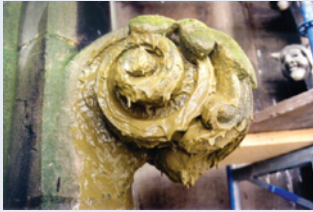
The masonRE® B product is sprayed or brushed onto a wet substrate and allowed to dwell
