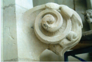
MasonRE® B breaks the bond between the carbon staining and the limestone or marble surface, leaving a clean substrate
