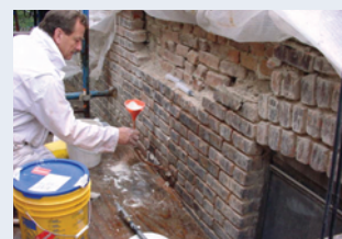
Mock up testing by Cathedral Stone on an exterior wall of the condominium building
