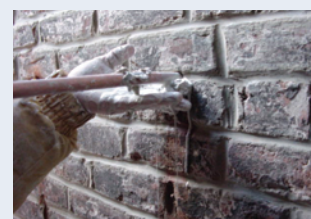
Installation of all-natural Jahn M30 injection grout provides structural stability
